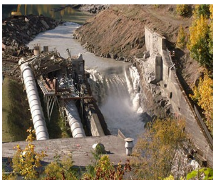
Lower Elwha Dam removal on October 24, 2011.
